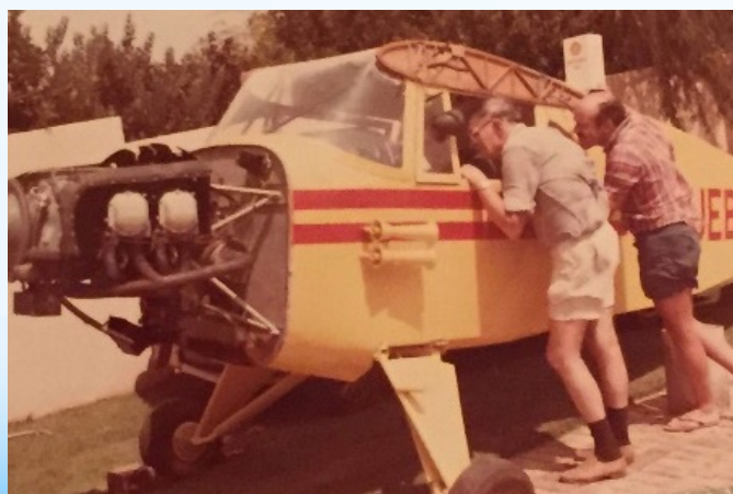
Fuselage covered, engine installed
